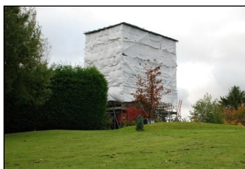
The mill today – shrouded in scaffolding
